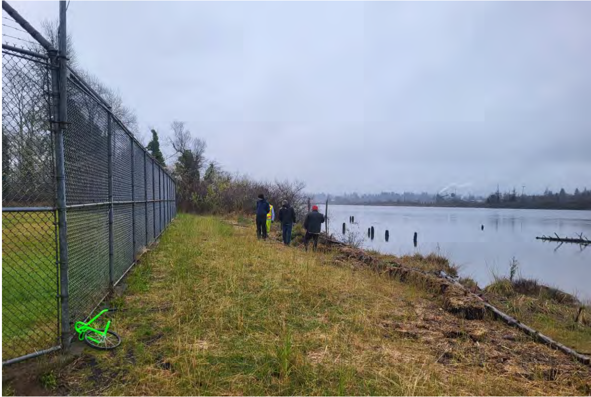
Figure 11. Distance between the project site shoreline and the Grays Harbor Juvenile Detention Center security fence. Timber piles near shoreline of project site. None of the alternatives propose impacts to the piles.
